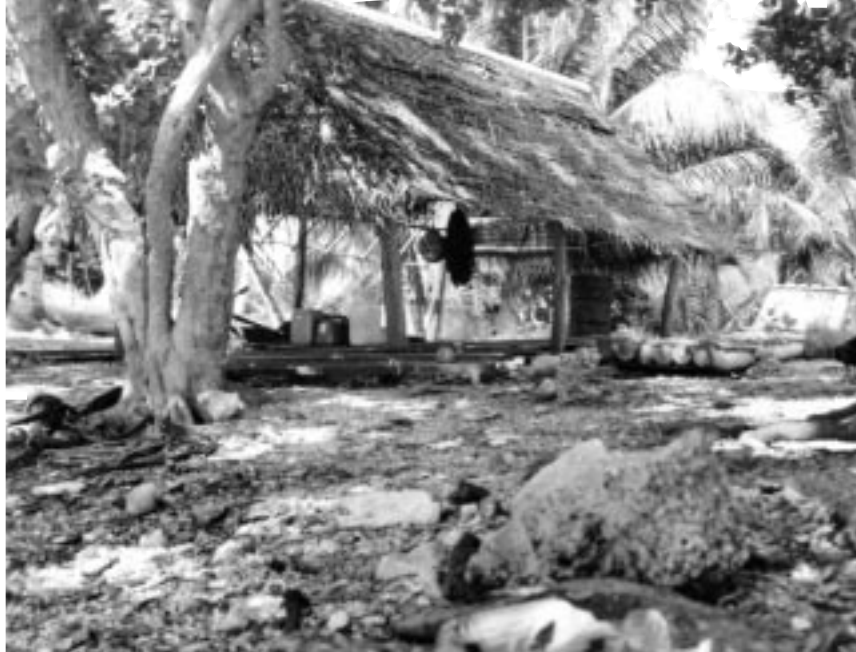
Figure 9. Boat house-shelter, Merir.
