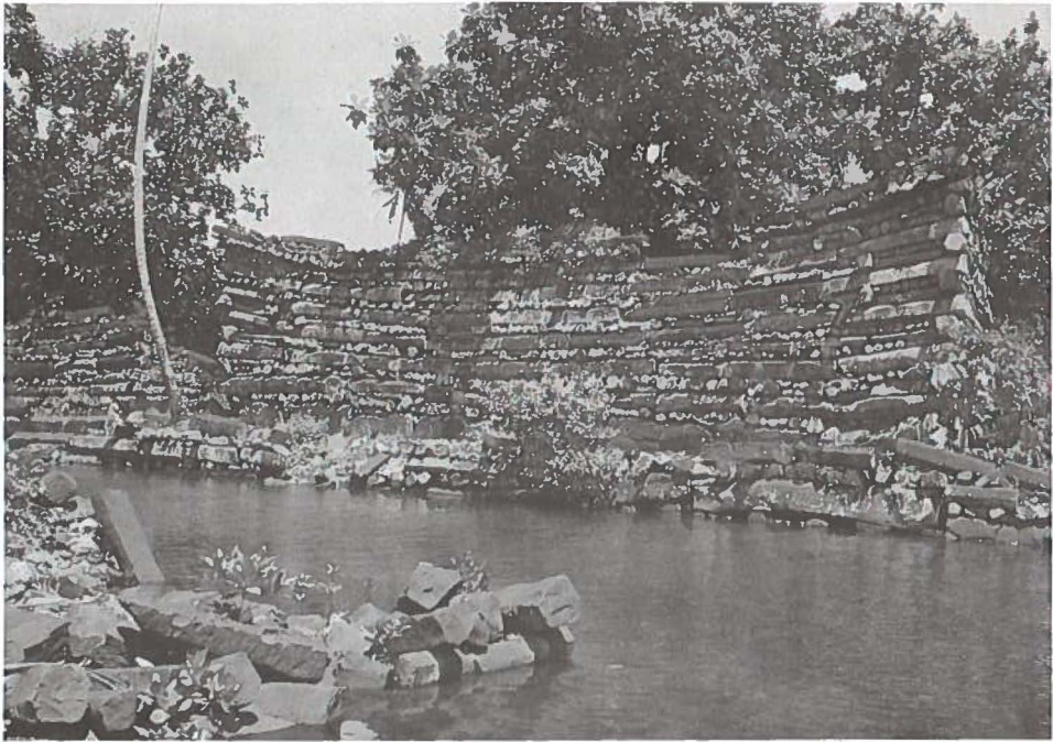
Figure 4. Photograph of west wall, Nandauwas islet, illustrating header-stretcher construction and corner treatment. Photo by Athens.
